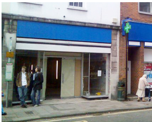
3 Bell Street, Henley before refurbishment
