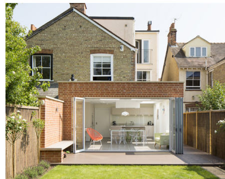
Successful contemporary extensions to traditional buildings in Watlington and London
