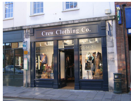
3 Bell Street, Henley after refurbishment
