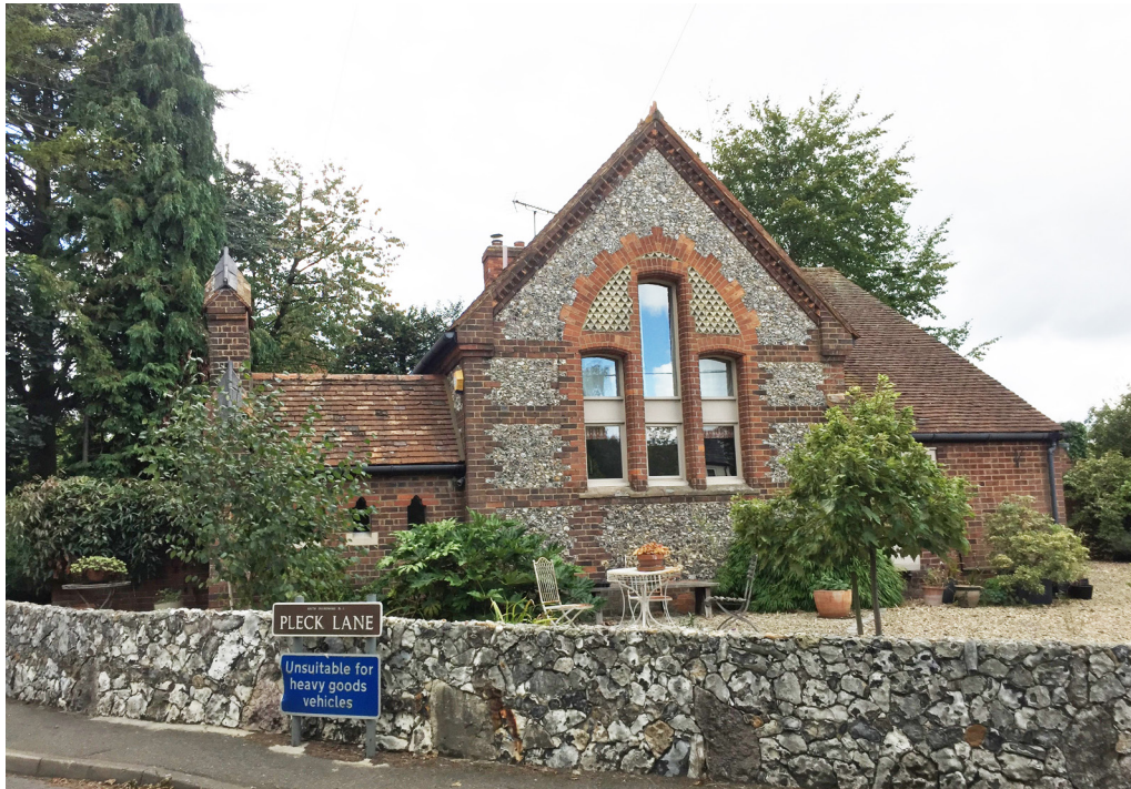
Conversion of an existing chapel in Kingston Blount
