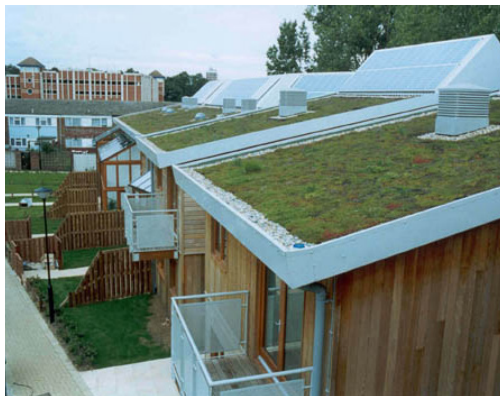
Example of an extensive green roof (Maidenhead)
