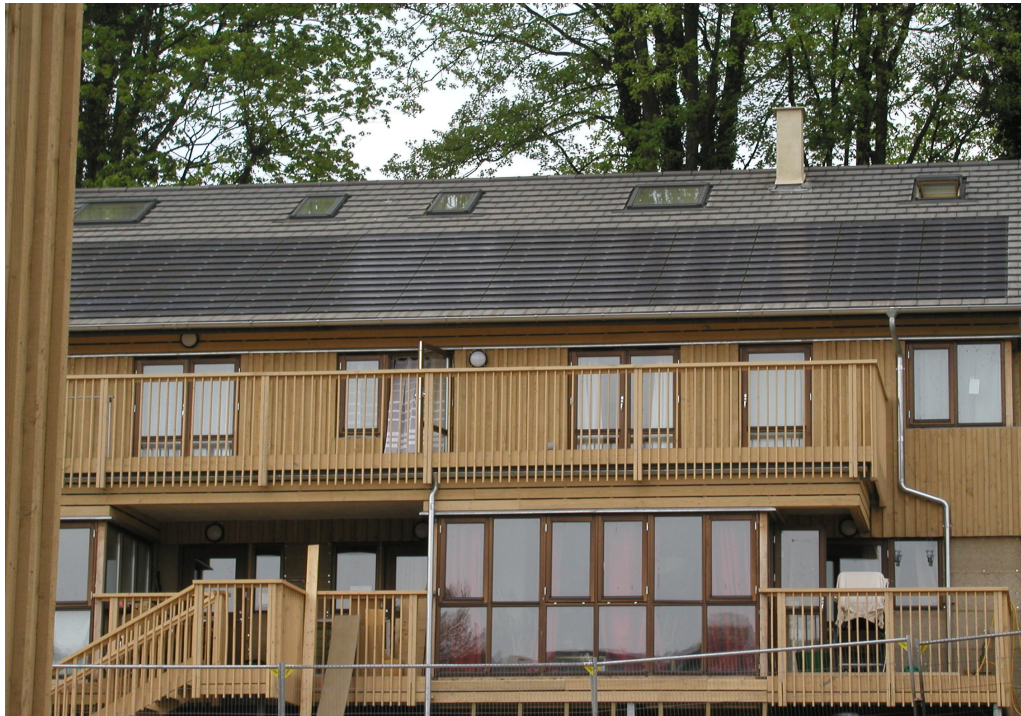
An example of solar roof tiles (Stroud, Gloucestershire)
